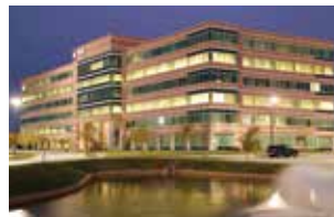
WireCo WorldGroup world headquarters, located in Kansas City, Missouri.
