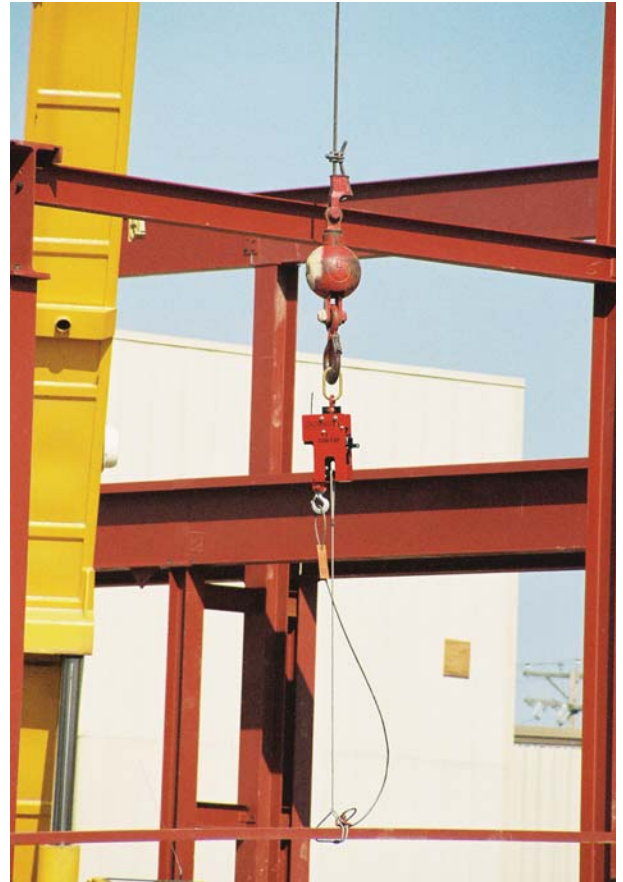
2.5 ton unit using a choker hitch
