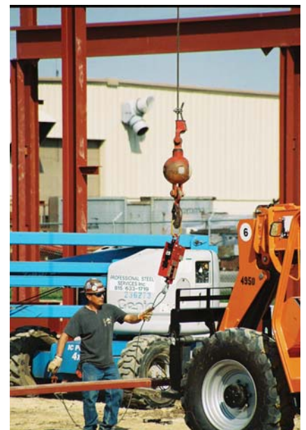
Setting header steel
